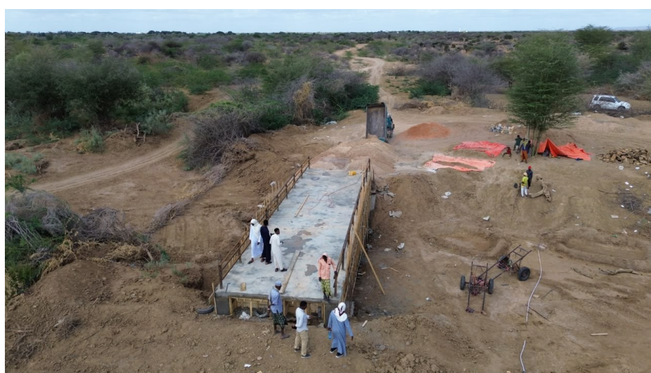
Figure 3. AARAN mini-bridge under construction, Bardheere (LLG activity photo).
